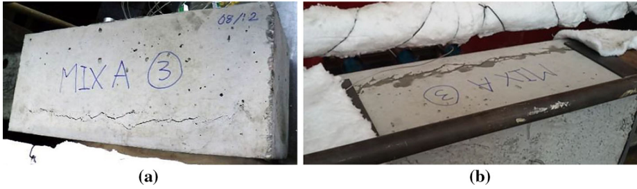
Figure 7. (a) Large crack on top of specimen Plain2-3. (b) Water/vapour escaping from the crack during test.
