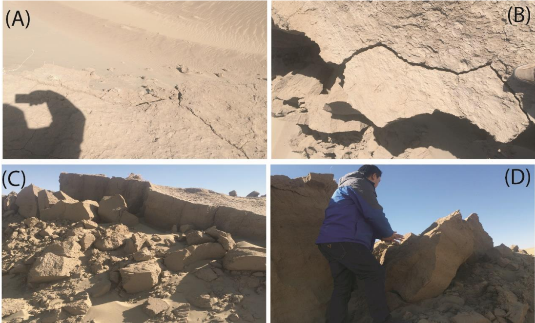
Figure12. Freeze-thaw induced fracture and side wall collapse during the Spring season in Gonghe basin blowouts
