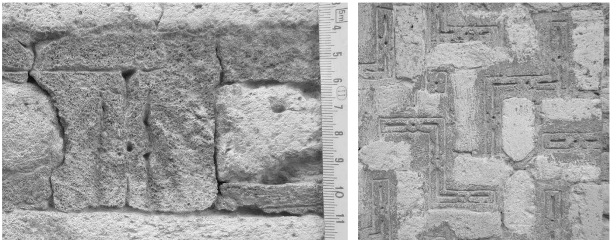
Fig. 9 – X-and-circle mortar incisions around the portal (L) and incised mortar patterns in the portal cavetto (R) of the Yūsuf ibn Kuthayyir tomb © R. McClary
