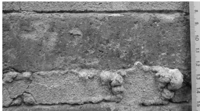
Fig. 33 – Kirk Kızlar tomb, Niksar; exterior salt efflorescence damage © R. McClary
