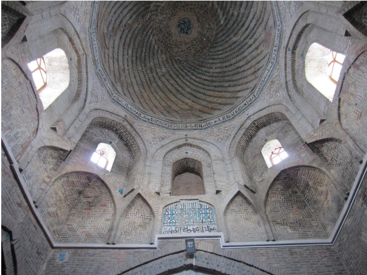
Fig. 12 – Malatya Great Mosque (645/1247); large structural brick muqarnas cells in maqṣūra dome squinches © R. McClary
