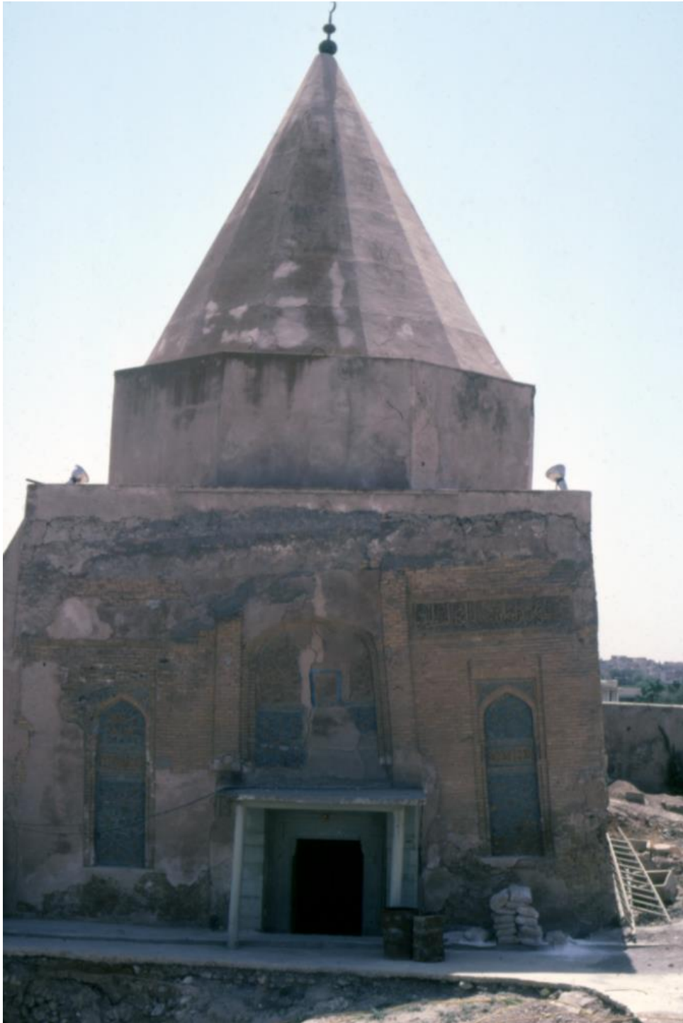
Figure 3 Northwest façade of the mashhad of Yahyā ibn al-Qāsim in 1983 © Yasser Tabbaa Archive, Aga Khan Documentation Center at MIT
