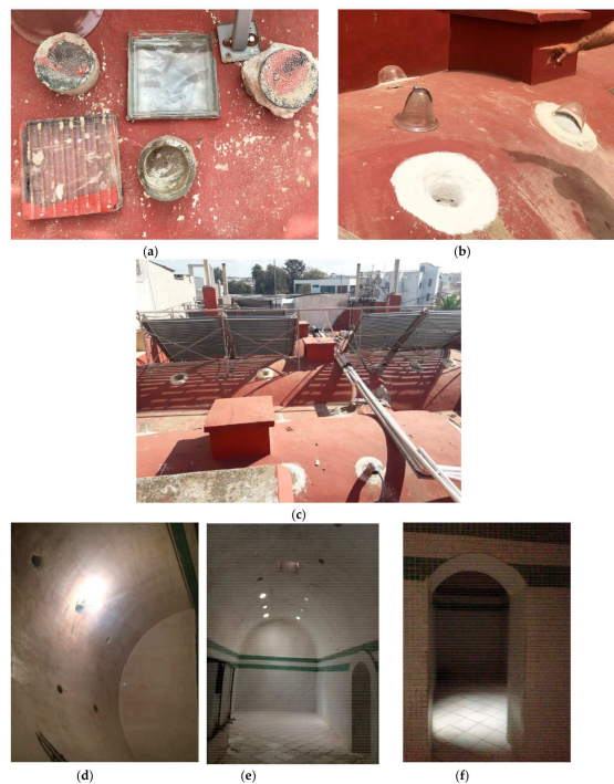
Figure 12. The roof of Hammam Rjafalla: (a) Removing poor alternatives of oculi covers; (b) re-opening the oculi and placing the blown recycled glass caps; (c) solar panels over the warm room affecting indoor daylight measurements; (d) blocked oculi in the hot room; (e) vernacular daylight restored; (f) oculi natural light effect.
