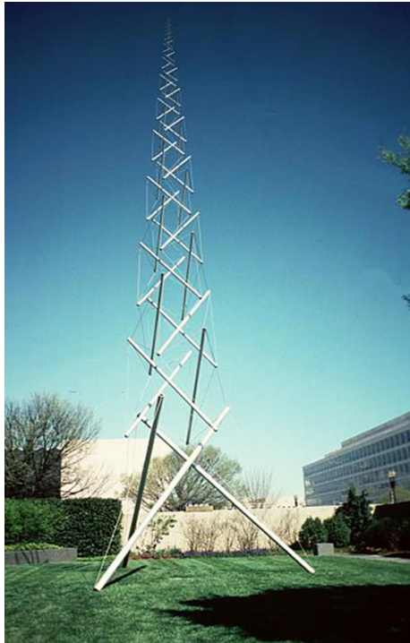
Fig. 1 Needle Tower (© 2002 Mary Ann Sullivan). Located at Hirshhorn Museum and Sculpture Garden in Washington D.C., USA. Made by sculptor Kenneth Snelson. Spatial construction [1]. 1991 reconstruction of the 1921 original. Made by Latvian artist Karl loganson, it is the very first tensegrity structure ever made
