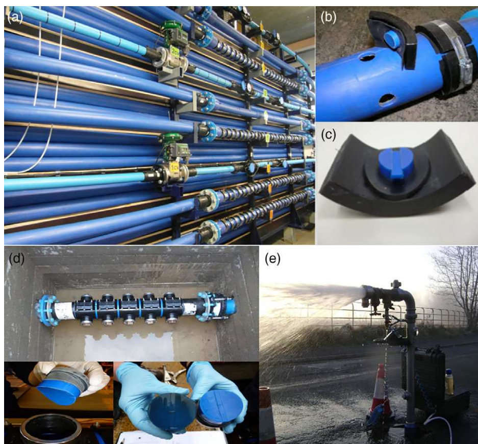
FIGURE 1 (a) Real-scale DWDS laboratory facility at Sheffield University, (b) PWG coupons are inserted along the pipe, (c) PWG coupons showing insert and outer part of the coupon. (d) Biofilm sampling devices used to sampling biofilm in situ during field work. (e) Flushing equipment used in real DWDS
