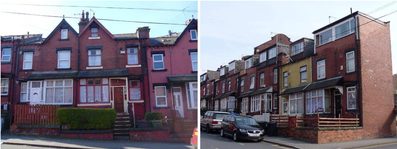
Figure 13. This row of blind backs in Character Area 2 has been particularly badly damaged. The photograph to the left shows houses where the design has seen little alteration. To the right, further along the row of the same block of houses, the impact of removing the original gable dormers and replacing them with dormers of varying mass, position, fenestration and material can be seen in the streetscape which has lost its uniformity and charm. ©Joanne Harrison.
