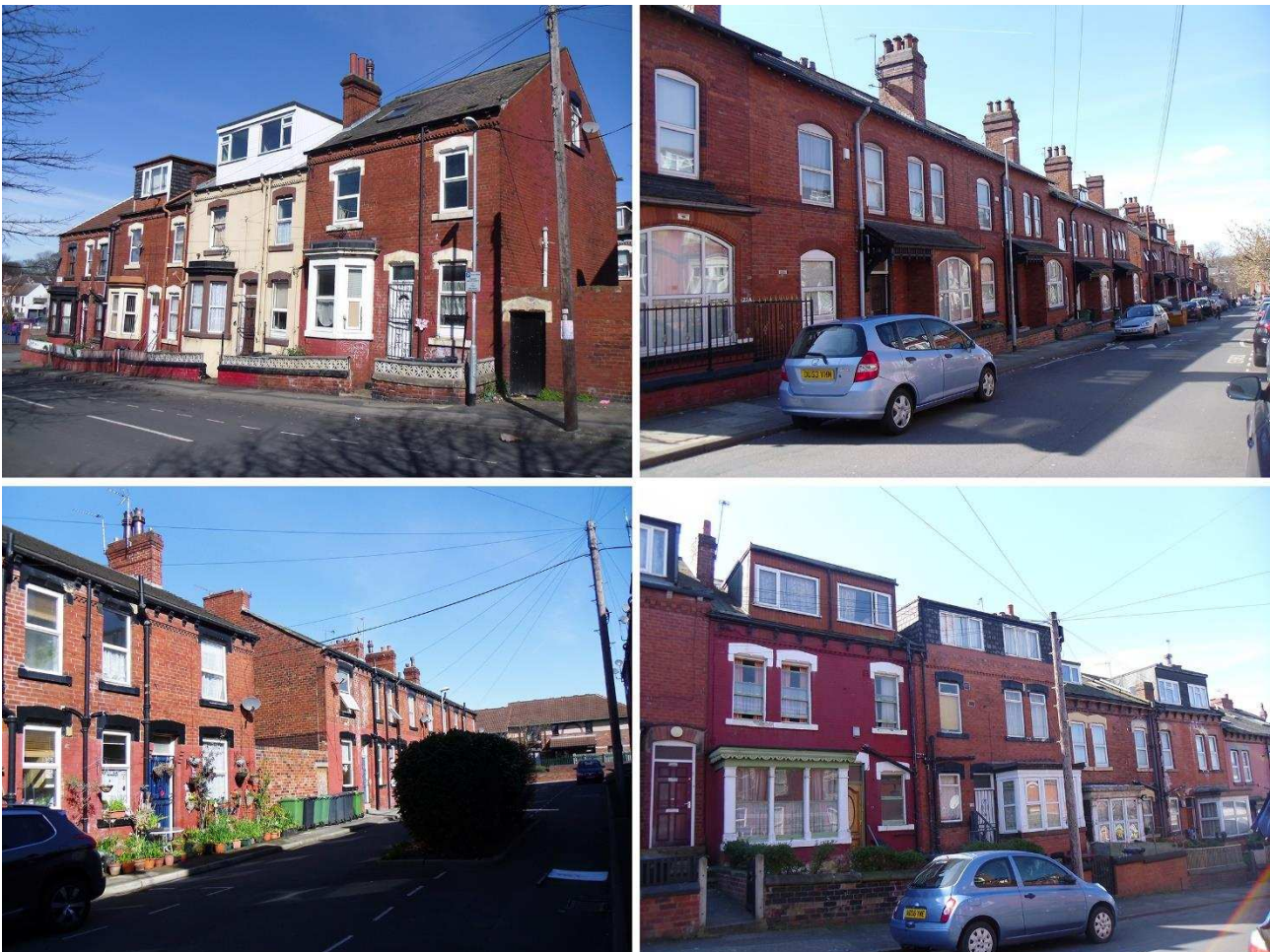
Figure 6. Character Area 2 is the most varied, and many of the designs include bay windows. The street-lined properties in the Edgwares (bottom left) are among the few in the area that do not have attics. ©Joanne Harrison.
