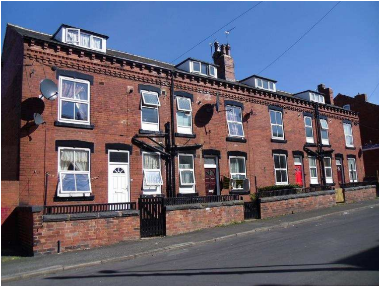
Figure 11. This block of houses has replacement windows which at least bear some resemblance to the original. In common with many houses they have an unattractive 'filler' panel installed to the bottom of the kitchen and bathroom windows in order to pro
