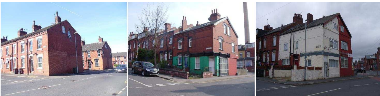
Figure 15. The house to the left has the most acceptable appearance as a house, but the shopfront has been lost in its entirety. By contrast, much of the shopfront is retained in the conversion in the centre image, and this is important to understanding the history and character of the area. The house to the right is one of the worst examples of shop-house conversions. ©Joanne Harrison.
