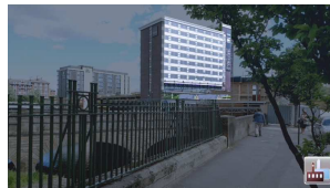
Fig. 16. The Metropolitan hotel after alignment.
