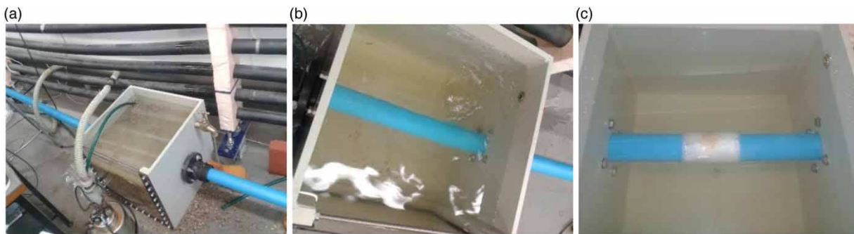
Figure 4 | Photographs of leaks in different backfill: (a) gravel media; (b) submerged; (c) geotextile fabric.
