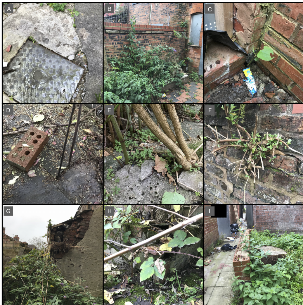
Figure 3 Photographs illustrating examples of the rating scheme that was applied. (A) Example of non-plant-based wear and tear to hard standing. (B) Rating '0'— B. davidii growing in a raised landscaping area, having no discernible impact on undamaged adjacent built structures. (C) Rating '1'— F. japonica emerging from existing cracks in paving at the base of a wall, causing no discernible impact away from baseline damage. (D) Rating '2'— F. japonica emerging from existing gaps in worn paving, while the gap has not been widened some mortar has been pushed aside. (E) Rating '3'— B. davidii growing out of a crack in worn concrete hardstanding, with additional cracks forming in the area. F. japonica visible in the background emerging from similar cracks in the hardstanding, also exacerbating existing damage but to a lesser extent. (F) Rating '3'— B. davidii growing out of cracks in worn brickwork, with additional cracks forming in the area. (G) Rating '4'— B. davidii growing out of cracks in worn brickwork. It has found its way between two structures and is facilitating the dilapidation of the wall and pushing out brickwork. (H) Rating '6'— B. davidii growing behind a small retaining wall and pushing some brickwork over. (I) The remains of a tree stump, which have destabilised the base of what remains of a dilapidated wall. Photos by M. Fennell.
