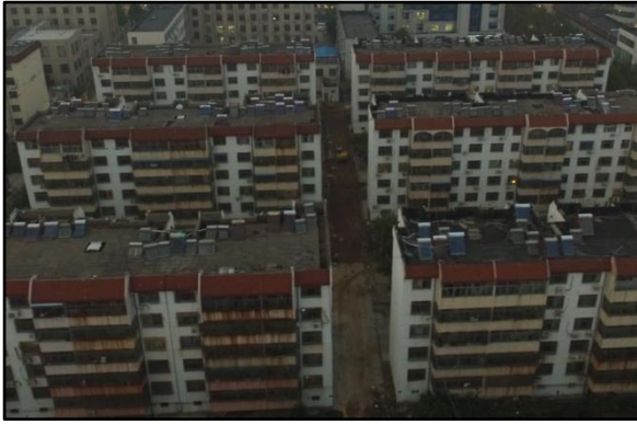
Fig. 5. Individually installed SWHs on the roof of residential buildings in Rizhao. (Photo taken by the first author, 2016)
