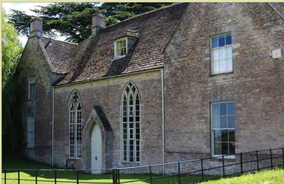
Figure 38: The Old Rectory, Ufford (formerly 'Uphall'). This was a medieval hall house; the wings on either side of the central hall were added later, and the windows are Victorian. The building is still in use as a house.
