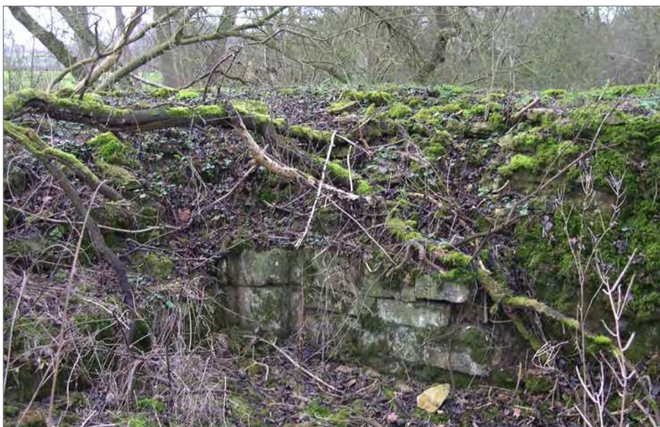
(c) Torpel Lodge remains: the interior southwest corner contains the sole remaining section of ashlar facing. The workmanship is of high quality and the courses vary between 8 and 11cm in height. The shaft was presumably the springer for rib-vaulting, forming the ceiling of the ground floor.
