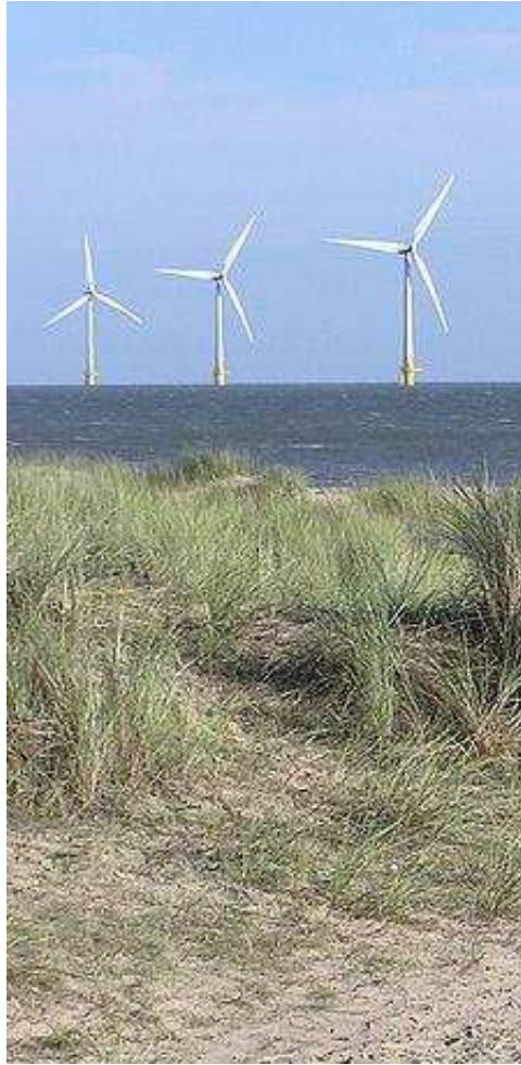
Figure A2: Example view of offshore wind project that is ~2 miles from shore in Great Yarmouth, England (Scroby Sands Wind Farm)
