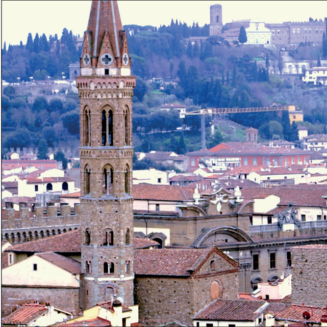
Figure 5. Bell tower of Badia Fiorentina, Firenze
