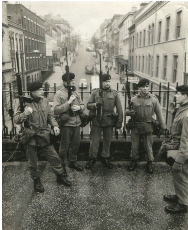
Figure 3. British Army occupation of the Walls, 1969 (Source: i.pining.com).
