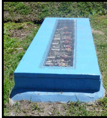
Photograph 2. New water connections at an informal settlement, fairly distributed by a natural leader
