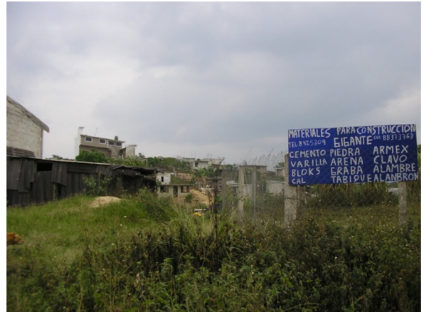
Fig. 13. Construction business in Esmerelda. Source: Melanie Lombard (2007).
