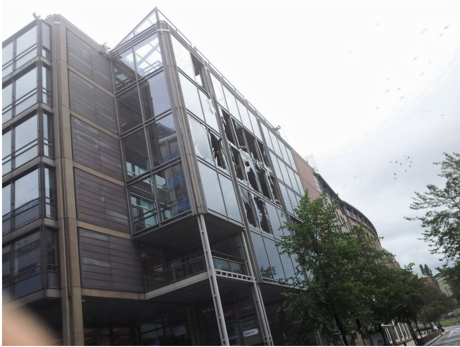
Figure 2: Window damage after the 2011 Oslo bombings (© Andreas Lunde/Demotix)
