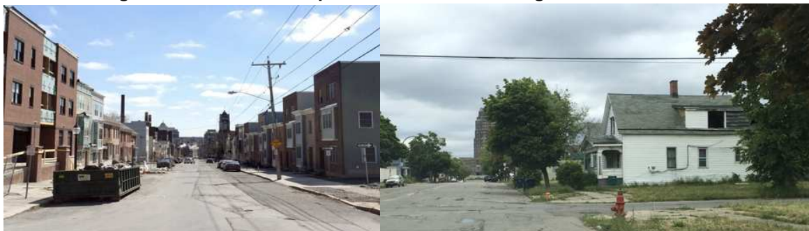
Left photo: Habitat for Humanity project courtesy of alloveralbany.com ; Right photo: author's own of the Eastside of Buffalo.
