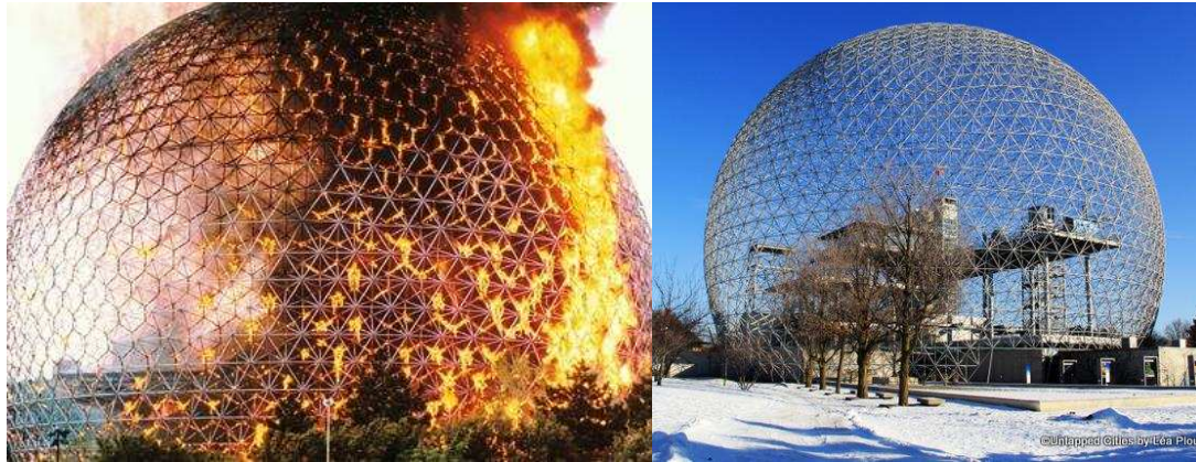
(a) During fire (b) After repair
