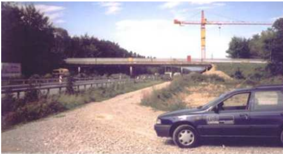
Figure 2: The Z24 bridge.
