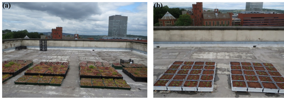
Fig. 1. (a) View of the test site before module installation on the 9th storey of the Education Building, University of Sheffield. (b) Installed green roof modules with Prunella vulgaris plugs planted. Aspect in both figures is facing north.
