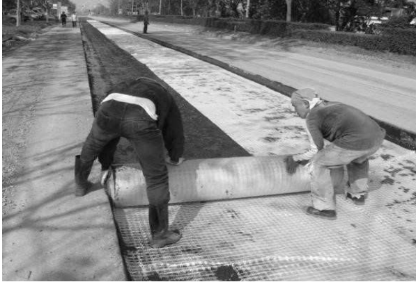
Figure 1. Photograph showing an installation of geotextile in a test section.
