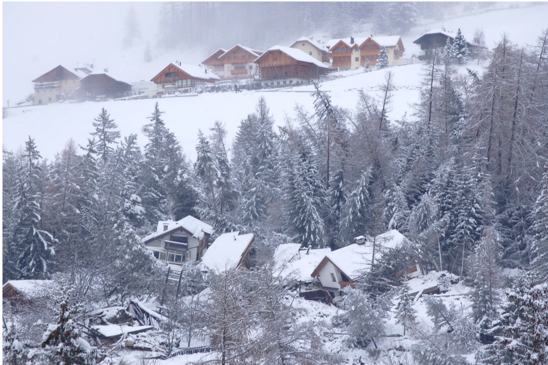
Figure 5: Photo of the landslide event in Badia in December 2012 Destroyed residential buildings in the foreground. Source: Photo taken by Christian lasio
