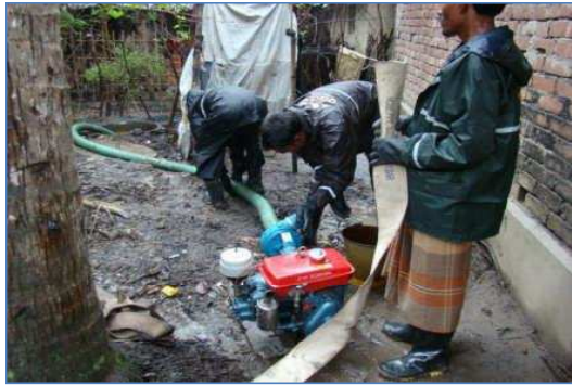
(c) Diesel pump
