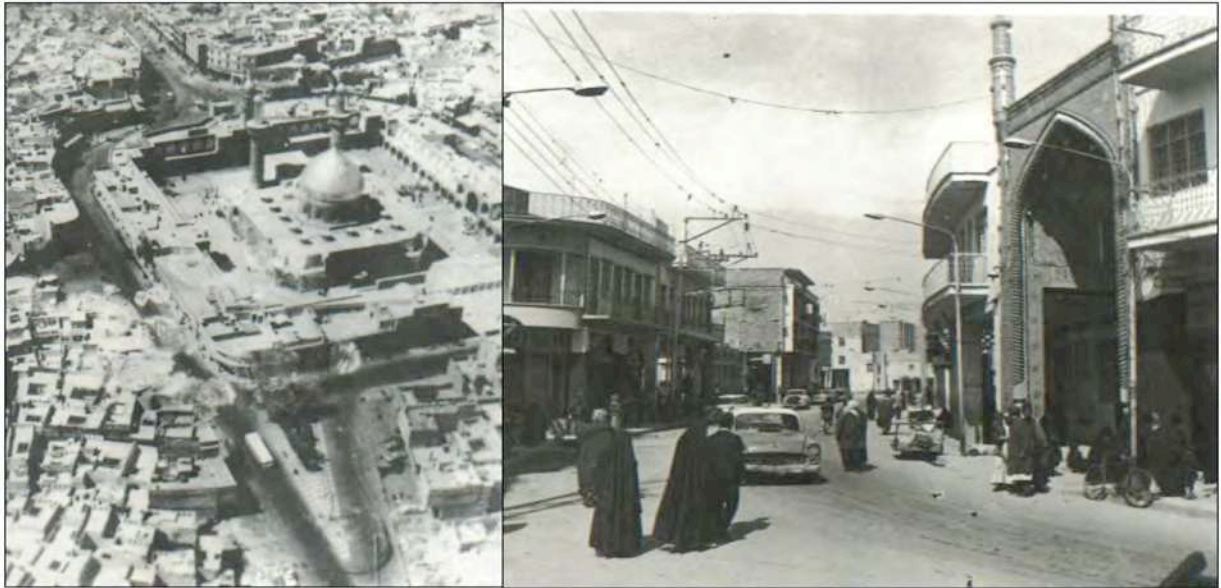
Figure 4. (Left) Holy Shrine after isolating it from the urban fabric, 1947 (Library of Hadara Abbasiya, 2005); (Right) Holy Shrine after isolating it from the urban fabric, 1947 (Dywan, 2011).
