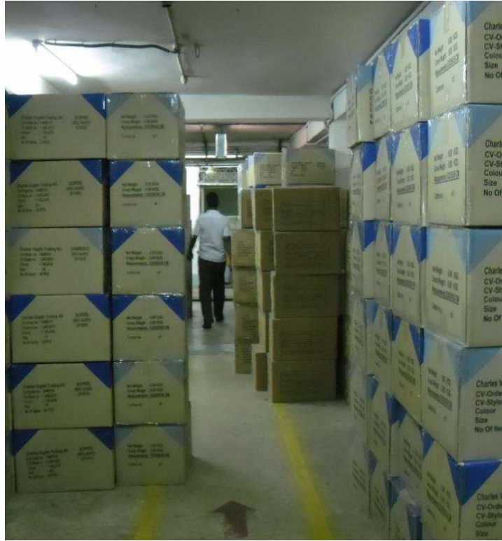
Figure-9: Soft factors: Exit corridor width meets regulation but reduced in practice.
