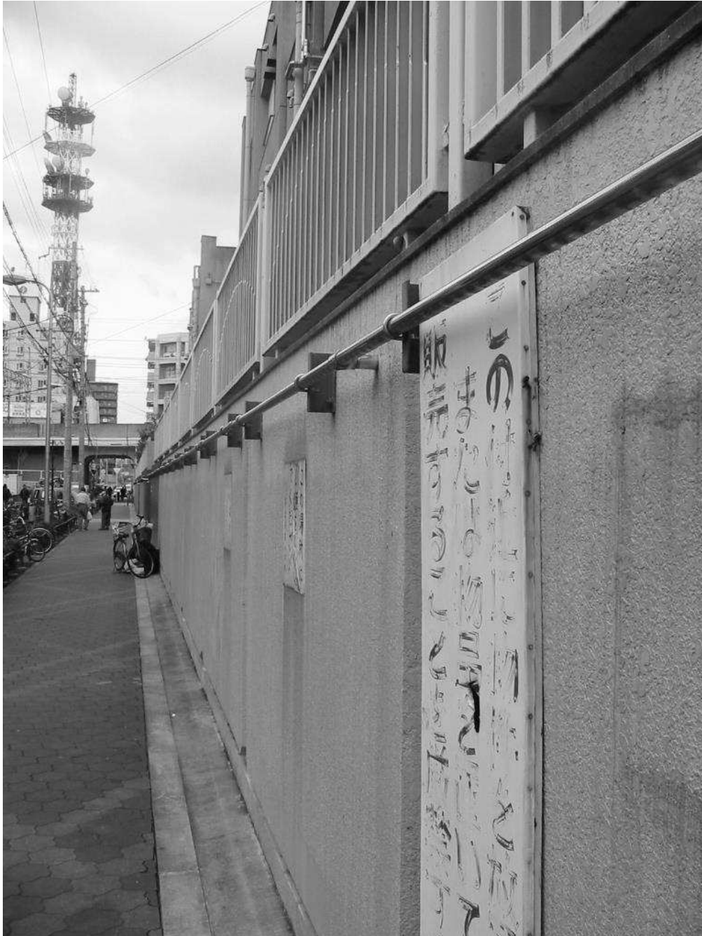
Figure 1: 'Bum-proof' walls. Shower-rail preventing homeless overnight street presence, Osaka (Source: Author)
