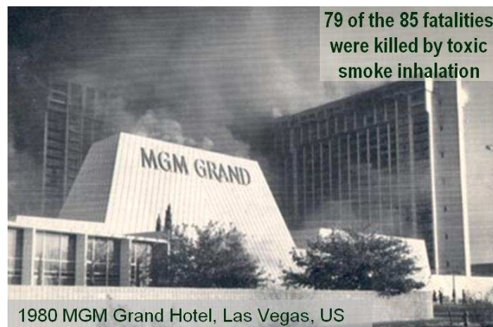
Figure 5: Picture of the MGM hotel during the fire showing the smoke dispersing from various areas in the building (Clark County Nevada Fire Department, 2010).
