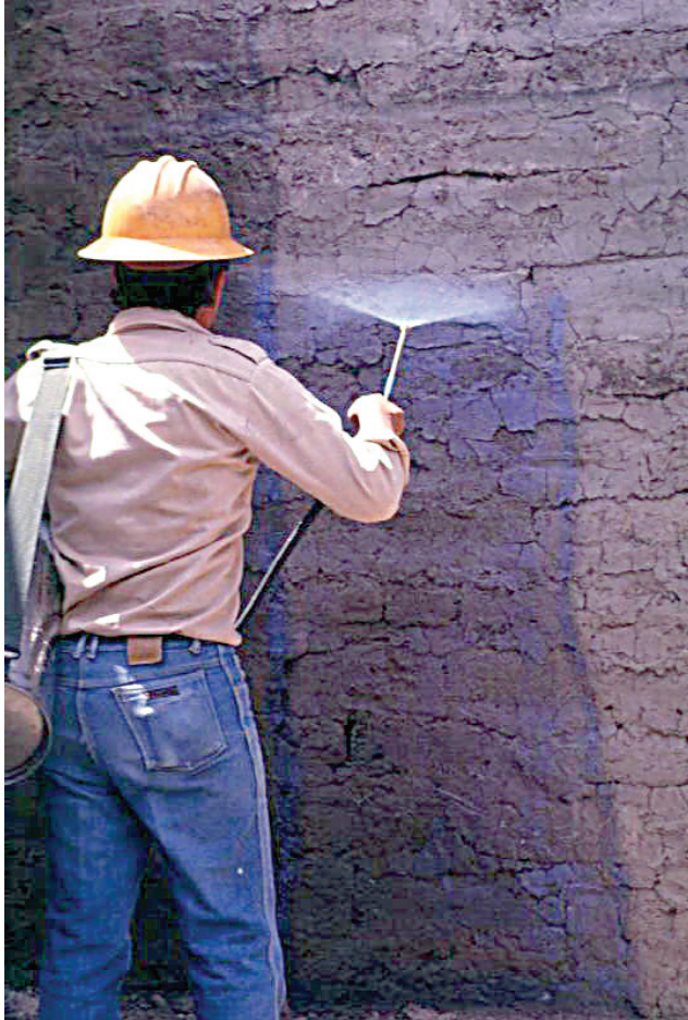
A sprayman coats houses, inside and out, with a slow-release insecticidal paint. The paint improves the appearance of the houses and is a relatively low-cost aid in helping to eliminate the triatomine bugs, the vectors of the parasites which cause Chagas Disease, 2002. WHO/TDR
