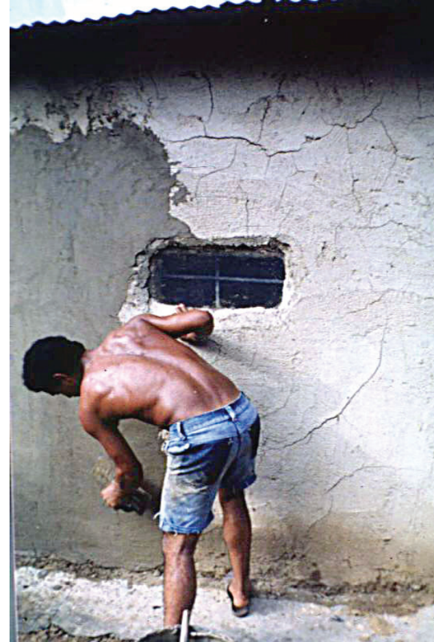
A man smooths plaster over cracks in the walls of his house. The cracks provide ideal habitats for the triatomine bugs that transmit the parasites which cause Chagas disease. 2002. WHO/TDR
