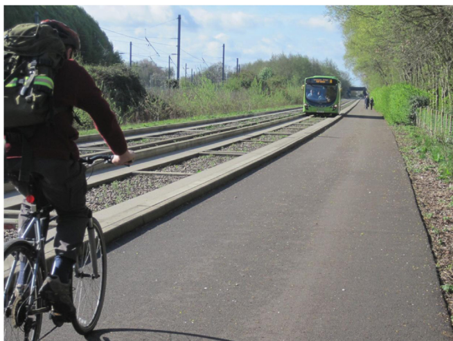
Fig. 1. The Cambridgeshire guided busway.
