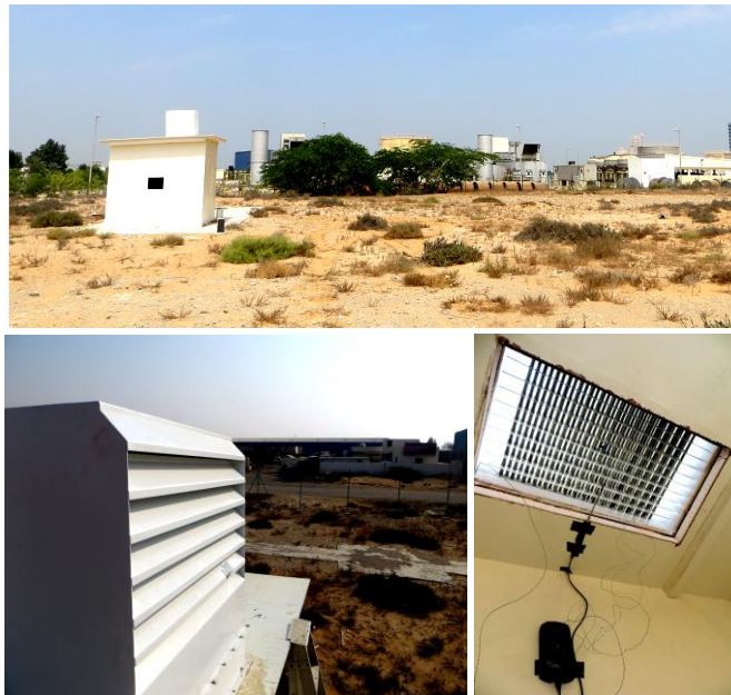
Figure 6: Test site in Ras Al-Khaimah (top) wind catcher mounted on the roof (bottom left) measurement setup (bottom right).
