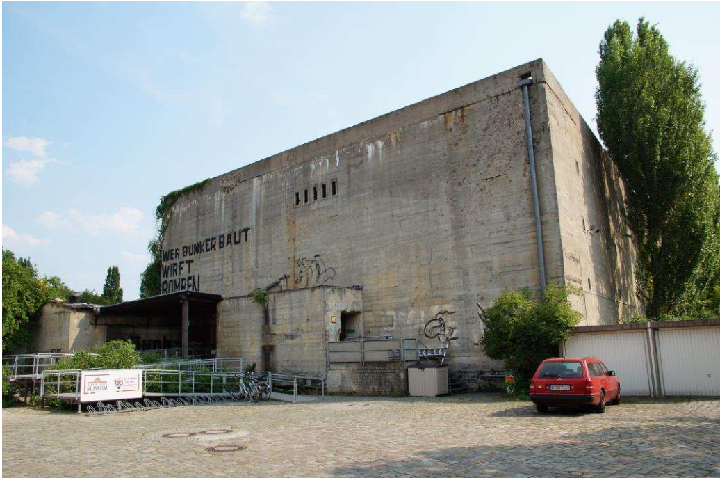
Illustration 1: Bunker at Anhalter Bahnhof, Berlin, B.R.D.: “ Wer Bunker baut wirft Bomben ” (He who builds bunkers, throws bombs).
