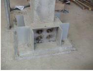
Figure 7: Steel foundation box
