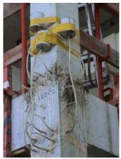
Figure 8: Injection of resin into crack
