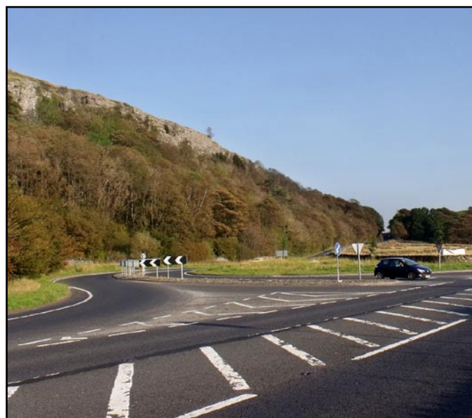
Figure 2: Giggleswick Scar North, looking east towards Buckhaw Brow along the line of the B6480 road (photo: P Murphy).
