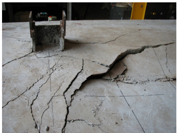
b) Compressive ring failure
