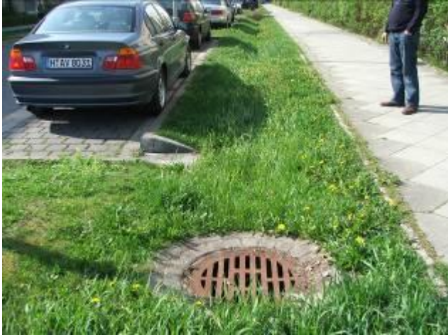
Mulden Rigolen providing street drainage in Kronsberg, Hannover
