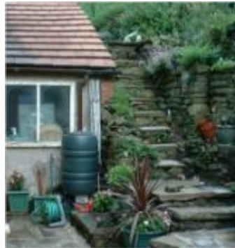
Typical water butt draining a roof
