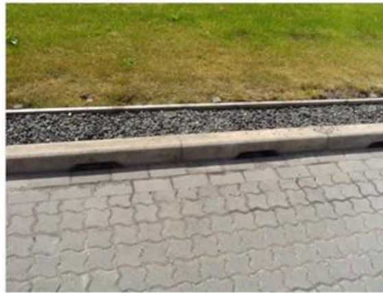
Filter Drain at J4M8 Industrial Estate, Scotland (University of Abertay)
