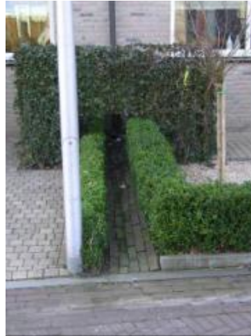
Roof drainage running into street gutter in Enschede (Mick Parr)
