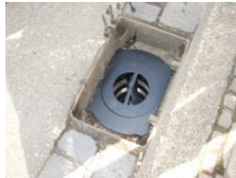
German gulley pot with "Innolet" cartridge filter
