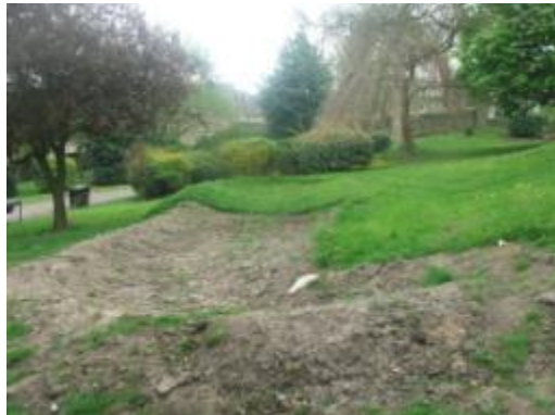
Swale under construction in Devonshire Park, Bradford
