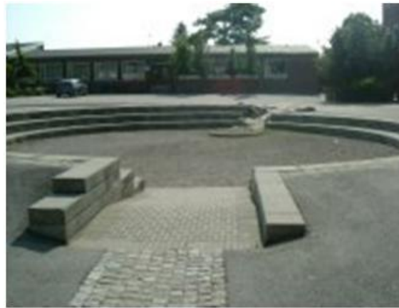
Detention Basin at Malmo (Virginia Stovin)
