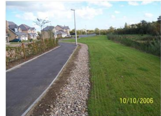
Filter Trench off-road, Scotland (University of Abertay)
