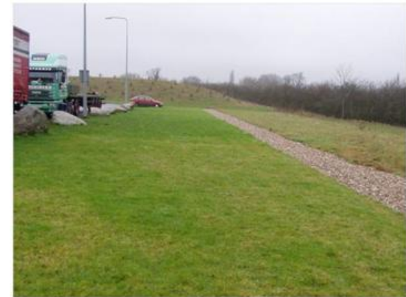
Filter Strip followed by a Filter Drain at Hopwood England
