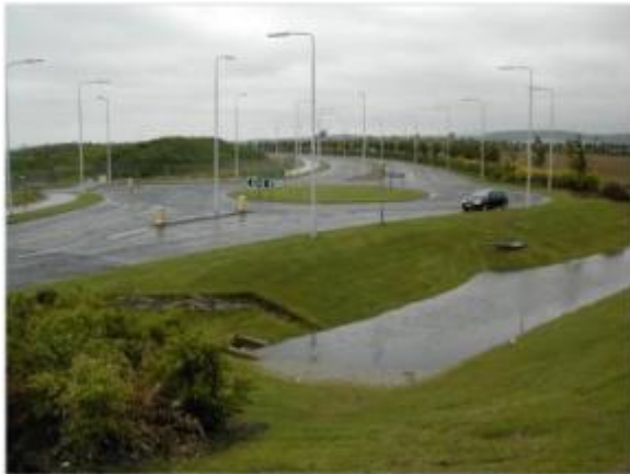
Roadside Detention Basin at DEX, Scotland (University of Abertay)
