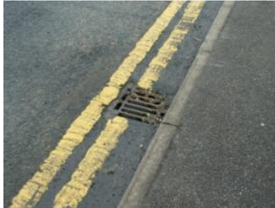
Gulley grate in Bradford
