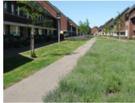
Estate scale rain garden (Bio-retention) in Utrecht
