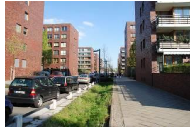
Mulden Rigolen providing street drainage in Berlin (Photo Harald Sommer)
