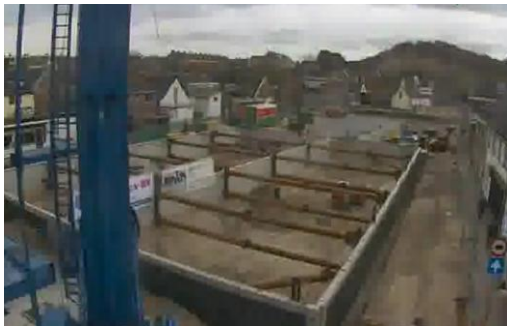
Concrete lined infiltration basin in dense urban area (Floris Boogaard)
