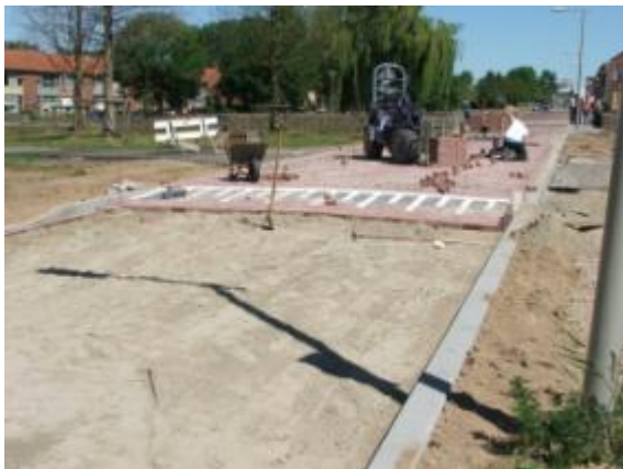
Permeable pavement construction in Arnhem
