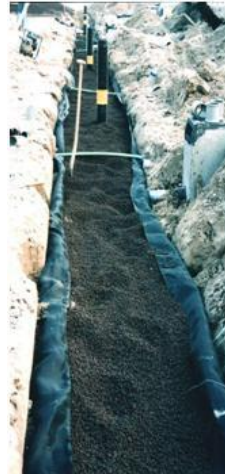
Infiltration trench under construction in the Netherlands
