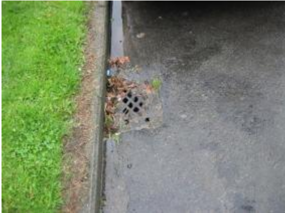
Gulley grate in Hull (Chrichton 2007)
