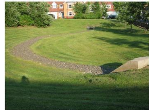
Detention Basin with curved flow path for attenuation and to hold the water for long time. Stirling, Scotland (University of Abertay)
