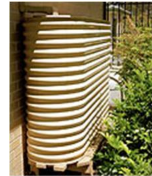
Australian large scale water butt for rainwater harvesting (Tony Weber)
