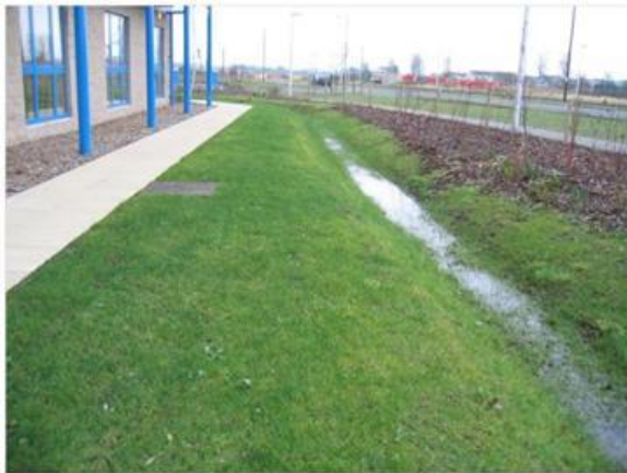
Filter Strip followed by a Swale in Dundee, Scotland (University of Abertay)
