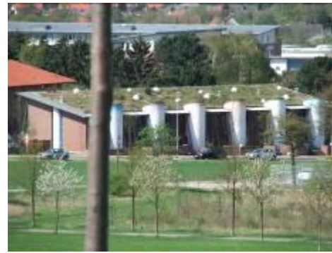
Green roof in Kronsberg, Hannover
