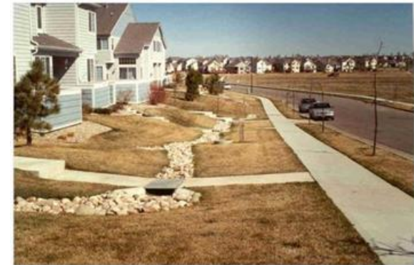
Filter Drain at Residential area at Fort Collins, USA (University of Abertay)
