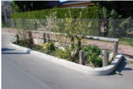
Street scale rain garden in Berlin. The water enters the rain garden through a gully (Harald Sommer)
