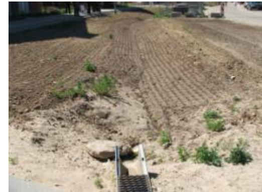
Swale under construction in Arnhem
