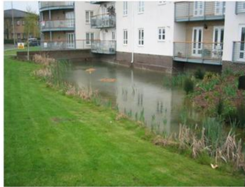
Retention Pond against the buildings in Tewkesbury, England (University of Abertay)
