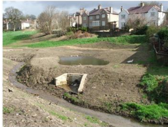
Constructed wetlands for water quality purposes at Bradford prior to planting
