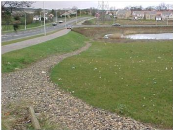
Filter Drain near Linburn Pond at DEX, Scotland (University of Abertay)
