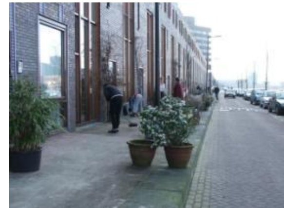
Permeable pavement reinstatement after utility works
