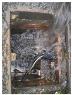
c) Flow entering gulley when grate raised
