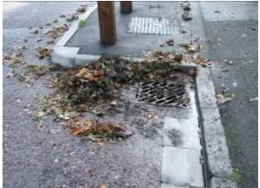
b) A larger grate but with small openings with a propensity to block
