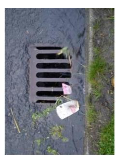
b) Flow bypassing gulley
