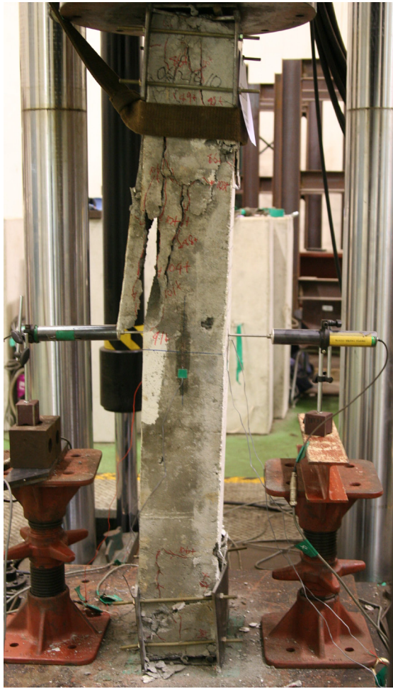
Fig. 7. Failure mode of column specimens
