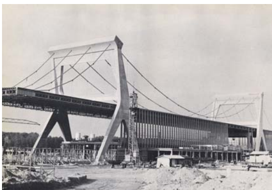
Fig. 3 The Burgo paper mill in construction, 1961
