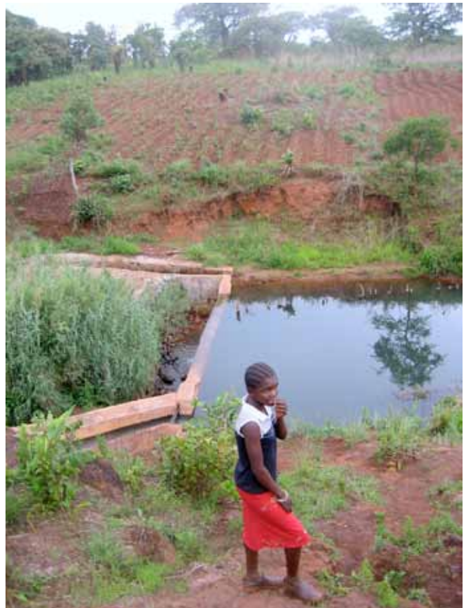
The beginning of the irrigation canal rehabilitated by Kansanshi Mine
