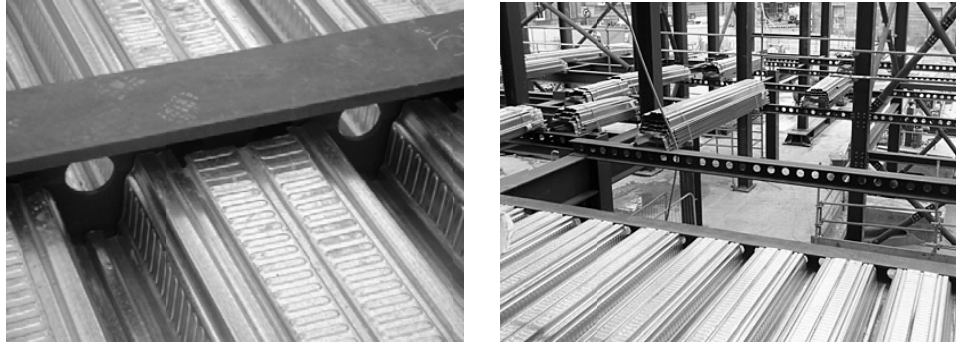
Figure 2. USFB construction adopted by Westok Ltd.
