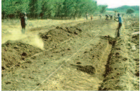
Figure 7.15 – Excavating the side ditch by hand in two stages using pegs, string lines and templates for guidance (photo courtesy: R. Petts).
