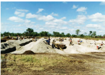
Figure 7.25 – Gravel being quarried for spreading as the surface running layer (photos courtesy: P. H. Bentall).
