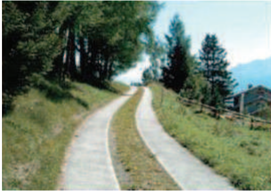
Figure 6.30 – Wheel strip paving (photo courtesy: Cook et al., 2013).
