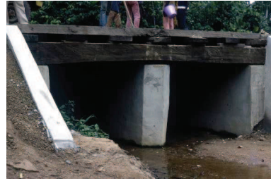
Figure 5.14 – Timber deck culvert (left) and timber deck bridge (above) nearing completion (photos courtesy: P. H. Bentall).
