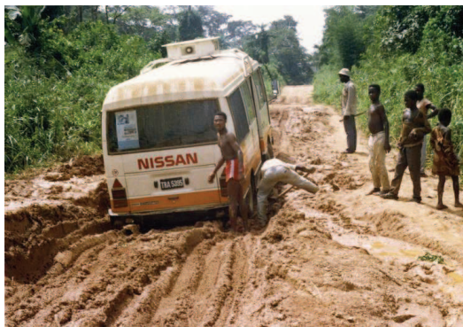
Figure 4.1 – Unsurfaced roads can become difficult to use in the wet season (photo courtesy: P. H. Bentall).
