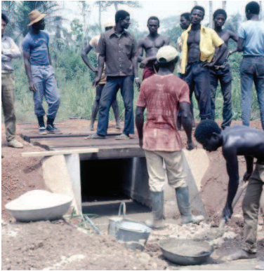
Figure 5.14 – Timber deck culvert (left) and timber deck bridge (above) nearing completion (photos courtesy: P. H. Bentall).
