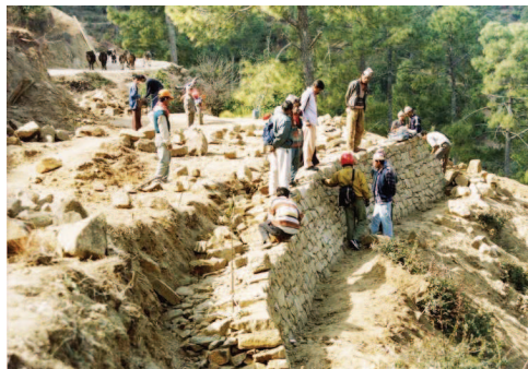
Figure 6.9 – Constructing a road with bends in mountainous Nepal (photo courtesy: P. H. Bental).
