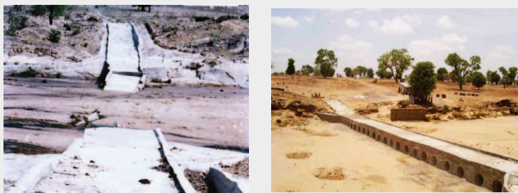
Figure A—The Dadiya River crossing pre and post construction.
