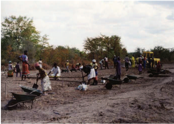
Figure 6.12 – Labour based earthworks (photo courtesy: P. H Bentall).
