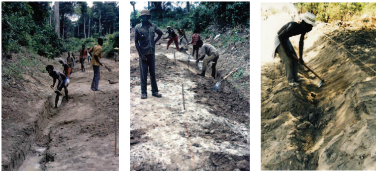
Figure 7.13 – Forming drainage side ditches by hand (photos courtesy: P. H. Bental).
