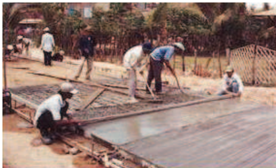
Figure 7.29 – Constructing reinforced concrete paving (photo courtesy: R. Petts).
