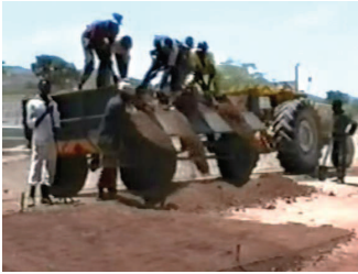
Figure 7.24 – Unloading and spreading gravel for the surface running layer (photos courtesy: P. H. Bentall).
