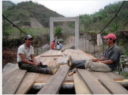
Figure B – Completing the new deck.
