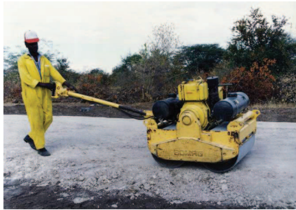
Figure 7.26 – Final compaction of the gravel surface layer (photos courtesy: P. H. Bentall).
