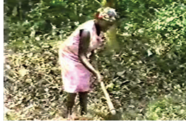
Figure 7.9 – Bush clearing and grubbing (photos courtesy: P. H. Bentall.)
