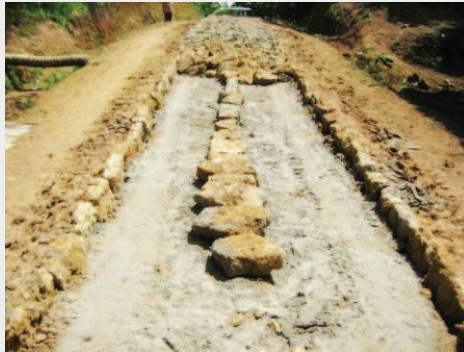
Figure A – ‘Telford’ road under construction in Nias.
