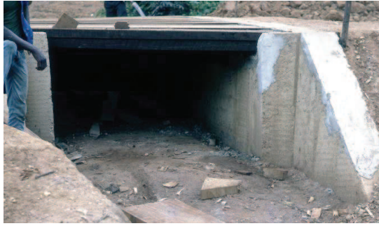
Figure 7.20 – Box culvert (photo courtesy: P. H. Bentall).
