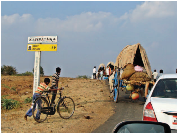
Figure 6.38 – Non-separation of motorised and non-motorised transport.
