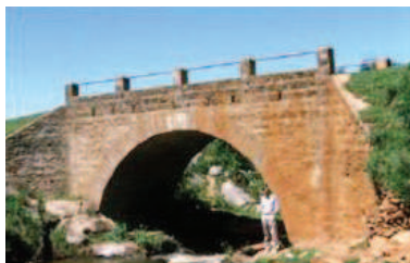
Figure 7.22 – Masonry arch bridge completed using local carpentry and masonry skills, and without lifting equipment (photo courtesy: R. Petts).
