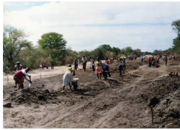
Figure 4.3 – Labour based road development projects under construction (photos courtesy: P. H. Bentall).
