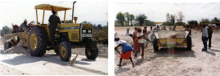
Figure 7.1 – Use of a tractor and trailer for haulage of gravel (photos courtesy: P. H. Bentall).
