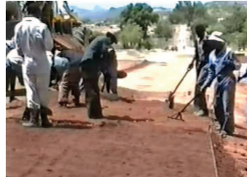
Figure 7.24 – Unloading and spreading gravel for the surface running layer (photos courtesy: P. H. Bentall).
