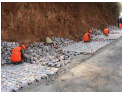
Figures 7.30 – Irregular cobble stone paving (left) and stone sets/pavé (right) (photos courtesy R. Petts).
