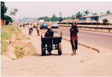
Figure 6.39 – Low cost separation of motorised and non-motorised transport (Overseas Road Note 21, © TRL, 2004).
