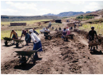
Figure 4.3 – Labour based road development projects under construction (photos courtesy: P. H. Bentall).
