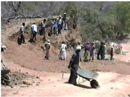
Figure 7.11 – Cutting material from an embankment to be used as fill (photo courtesy: P. H. Bentall).
