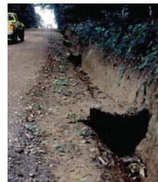
Figure 6.17 – (right) scour checks installed on site (photo courtesy: P. H. Bentall).
