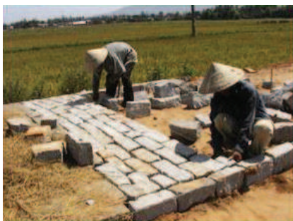
Figure 7.31 – Dressed stone paving using granite material, hand quarried and dressed (photo courtesy: R. Petts).
