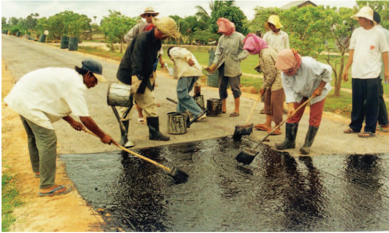
Figure 7.28 – Manual application of bitumen emulsion seal prior to chipping application (photo courtesy: R. Petts).
