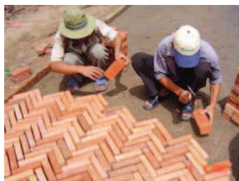
Figure 7.32 – Laying fired clay brick paving between previously placed edge restraints/kerbs (photo courtesy: R. Petts).
