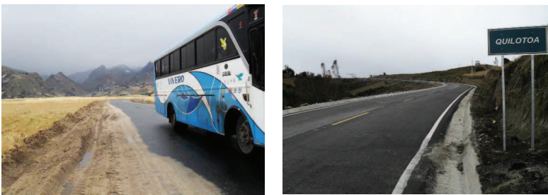
Figure 6.4 – Inadequate drainage (left) and upgraded drainage (right) (photos courtesy: A. McLoughlin).
