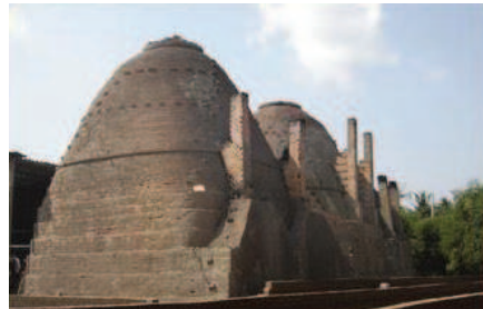
Figure 5.15 – Beehive or bell shaped kilns for rice husk firing of clay bricks suitable for road paving and structures (photo courtesy: Bach The Dzung).
