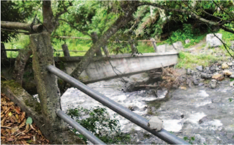
Figure 6.22 – The failure of this steel reinforced concrete bridge illustrates the need for appropriate design and construction (photo courtesy: A. McLoughlin).
