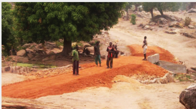
Figure B – Road approaches to a culvert close to completion.
