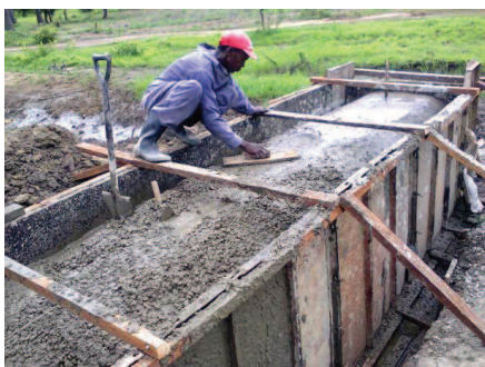
Figure 7.23 – Formwork being used to apply concrete to a corrugated steel pipe culvert (photo courtesy: K.Ogutu).
