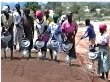
Figure 6.13 – Applying water to the road formation to achieve the OMC before compaction (photos courtesy: P. H Bentall).
