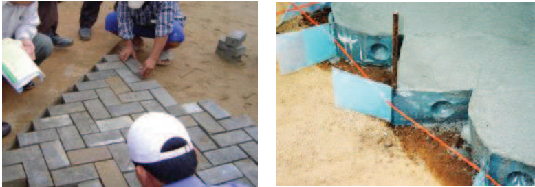
Figure 6.29 – concrete brick and geo-cell paving options (photos courtesy: R. Petts).
