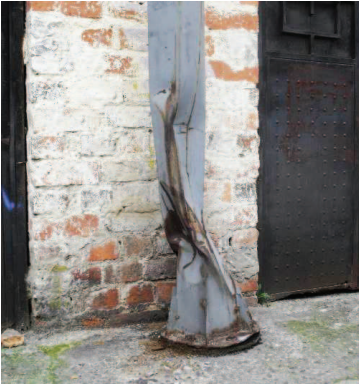
Figure 7.34 – Unrepaired street lighting columns and make-shift water crossings are only two examples of inadequate maintenance (photos courtesy: A. McLoughlin and P. H. Bentall).
