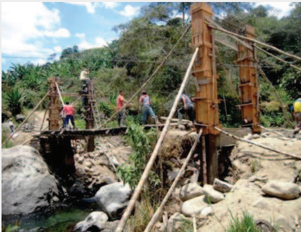
Figure A – The bridge during construction.
