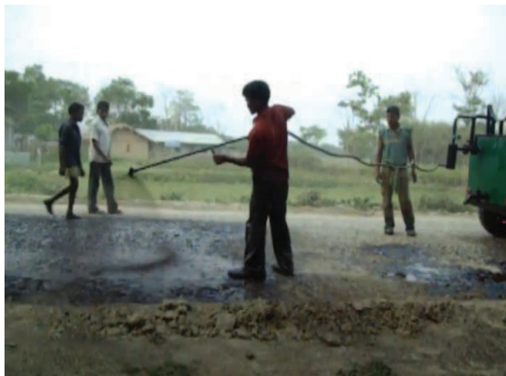
Figure 7.27 – Bitumen spray-lance in use.
