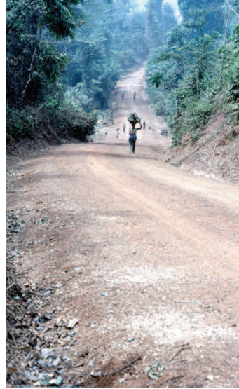
Figure 2.1 – This recently completed gravel road in Ghana makes travel to market much easier (photo courtesy: P. H. Bentall).
