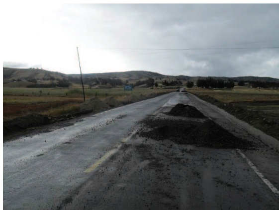
Figure 5.13 – This former gravel road has been recently upgraded to a bituminous standard (photo courtesy: A. McLoughlin).
