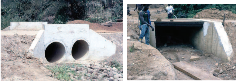
Figure 7.2 – Concrete double pipe culvert (left) and box culvert (right) (photos courtesy: P. H. Bentall).
