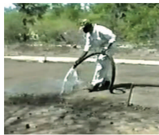
Figure 6.13 – Applying water to the road formation to achieve the OMC before compaction (photos courtesy: P. H Bentall).
