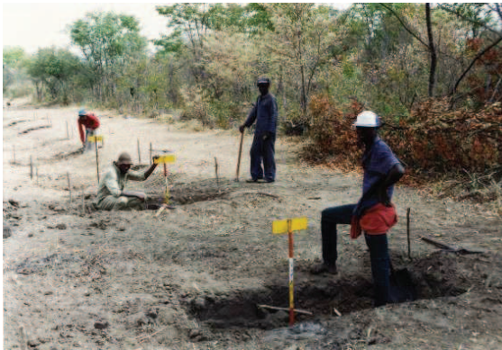
Figure 7.8 – (above and below) Setting out the vertical alignment on site using profile boards (photos courtesy: P. H. Bentall).
