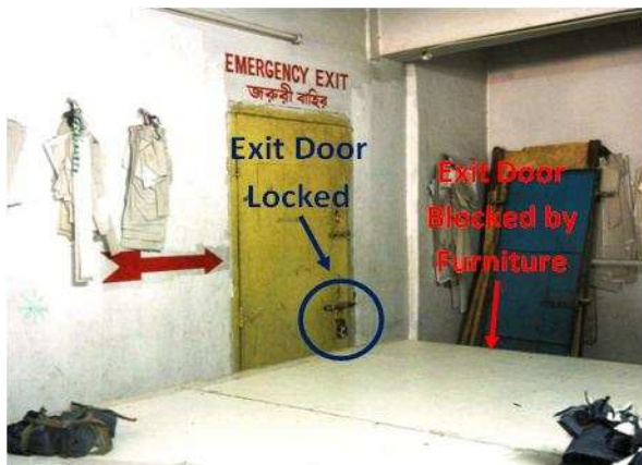
Fig 5: Exit Door Locked and Blocked by Furniture.
