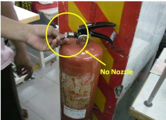
Fig 4: Fire Extinguisher with No Nozzle.
