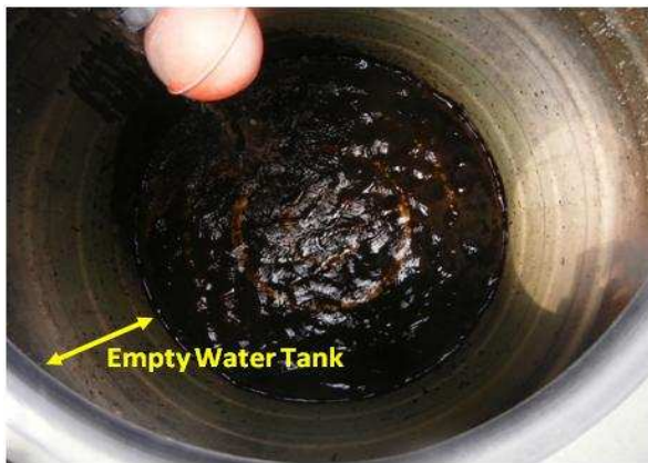
Fig 2: Empty overhead water tank for fire fighting.
