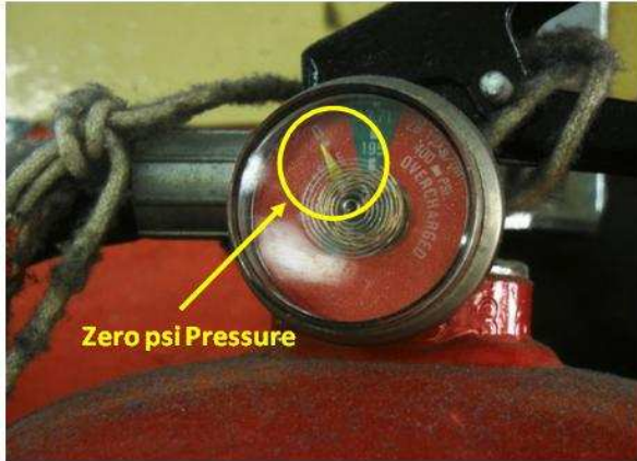
Fig 3: Fire Extinguisher with Zero Operating Pressure.
