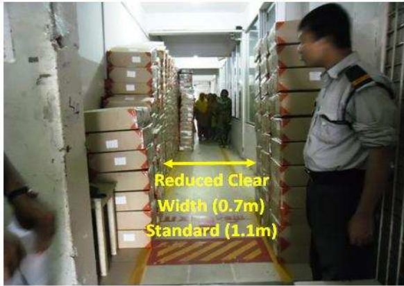
Fig 1: Clear width of an exit corridor reduced by piled up boxes.
