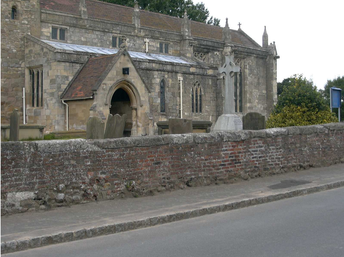
Fig 6: Lower courses of stone in south churchyard wall
