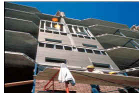
(b) Pre-cast concrete hollow slabs
