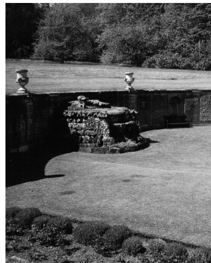
Figure 4. The old waterfall and pond in Parterre once supplied by water from another pond and 30-step cascade which in turn were fed by the T Pond
