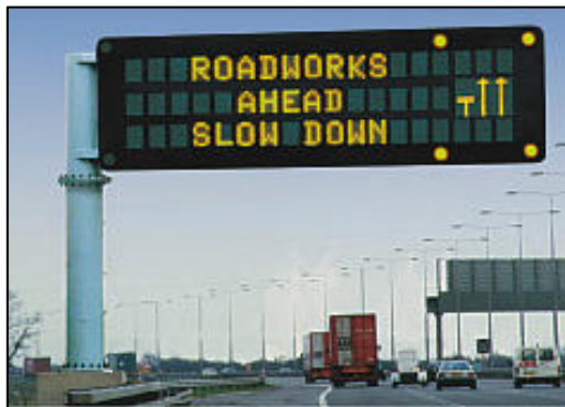
Figure 6: MS3 signs are being rolled out on the UK Motorway Network as part of the National Traffic Control Centre Project (source: The Highways Agency)
